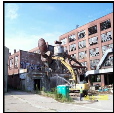
The City commenced building demolition in early 2007
