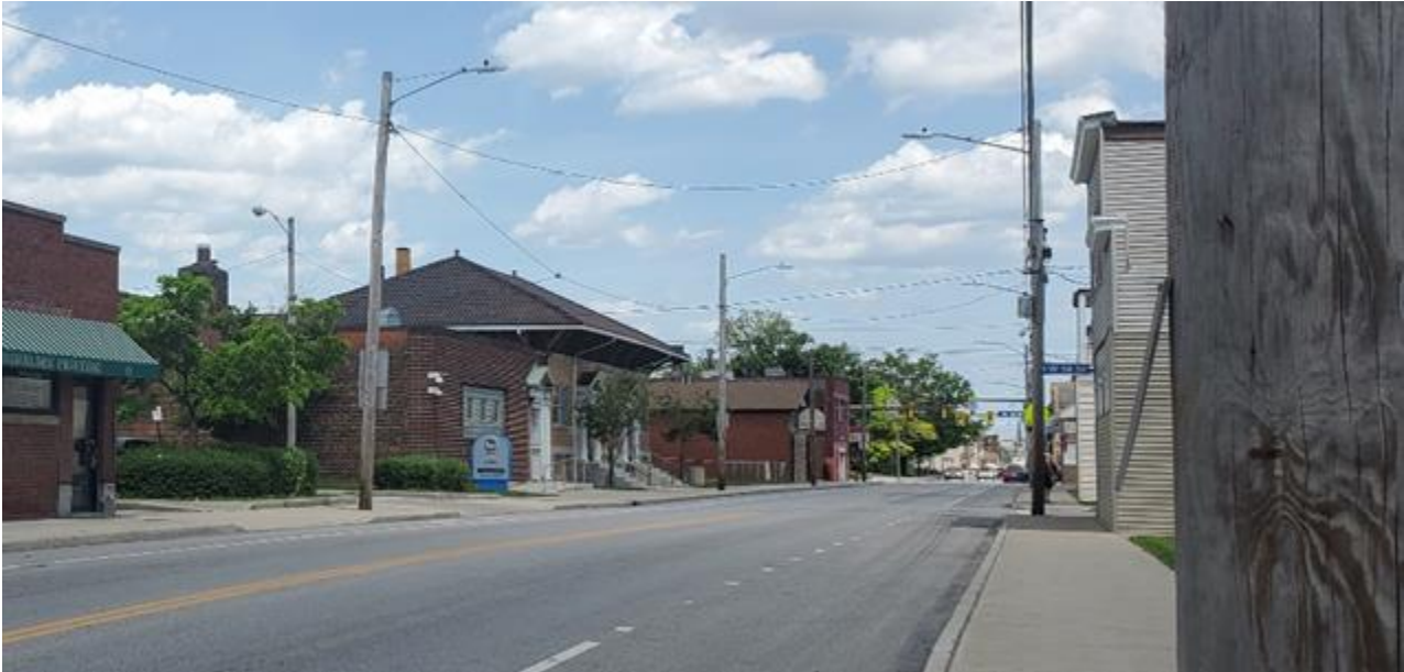
Photograph 2 - Front View from West
