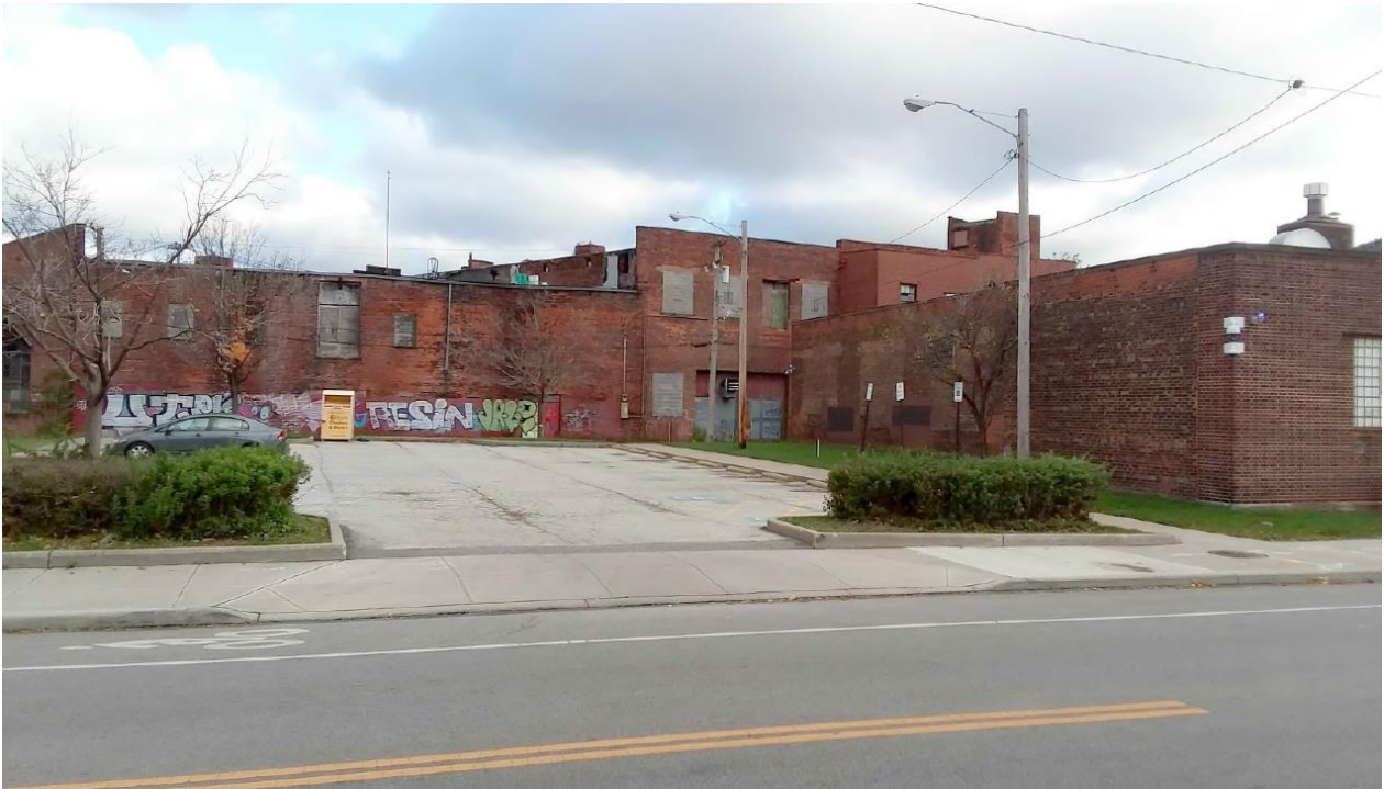
Photograph 3 - Parking Lot View from South
