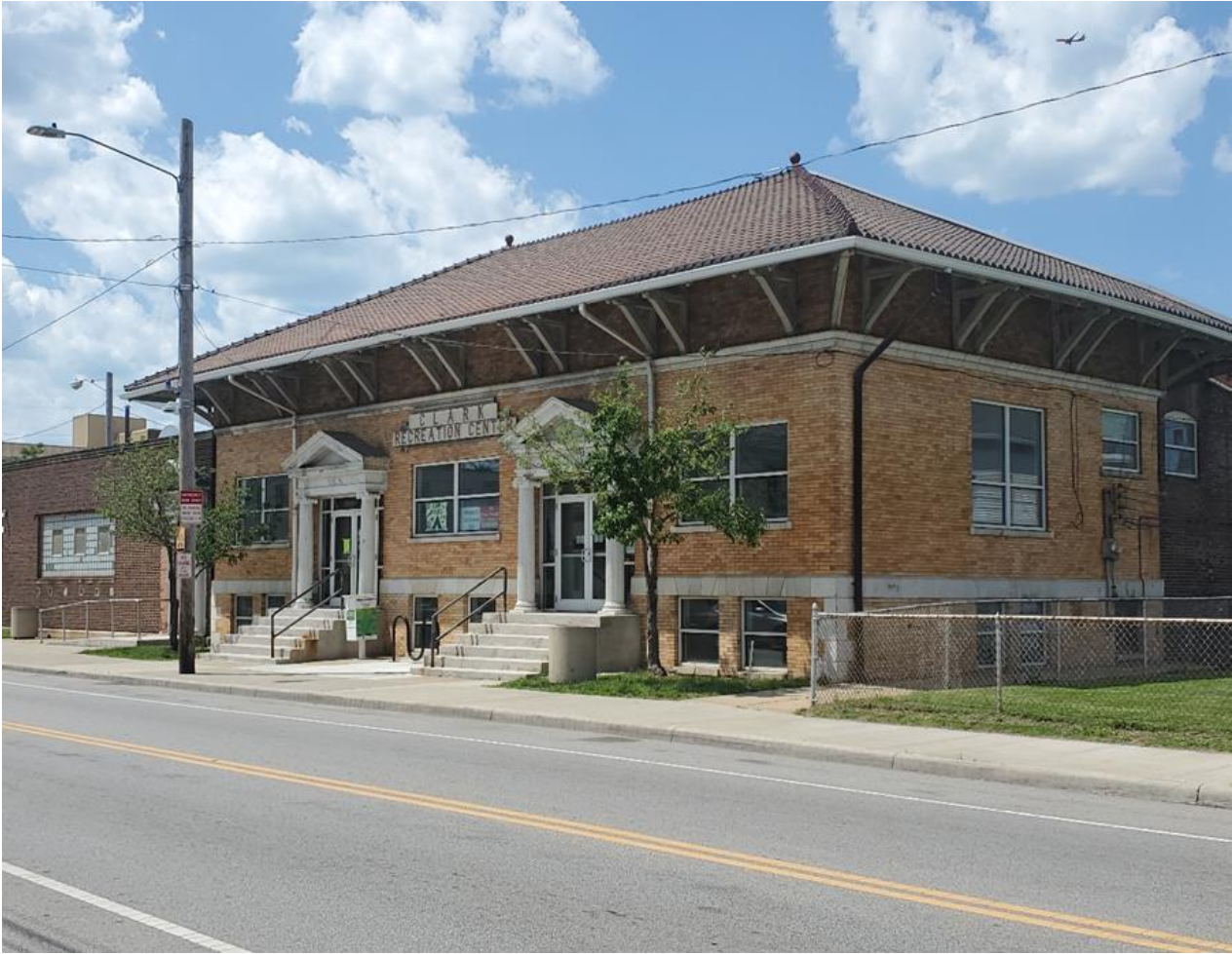
Photograph 1 - Front View from Southeast
