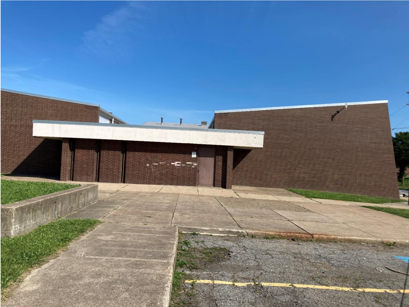
Photograph 2 - Side View from South (Parking Lot)
