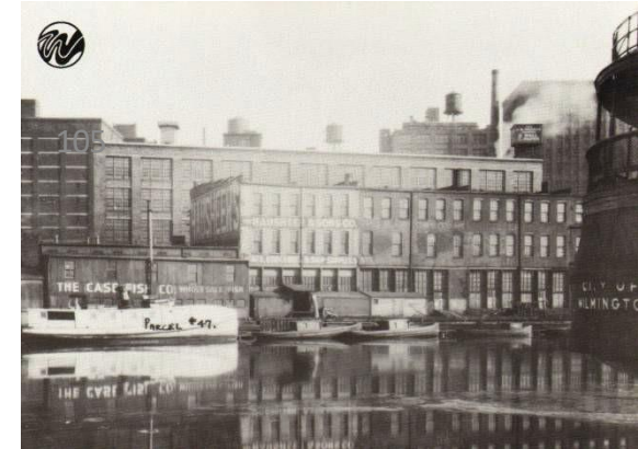
VIEW FROM RIVER C. 1920 THE HAUSHEER AND SONS BUILDING
