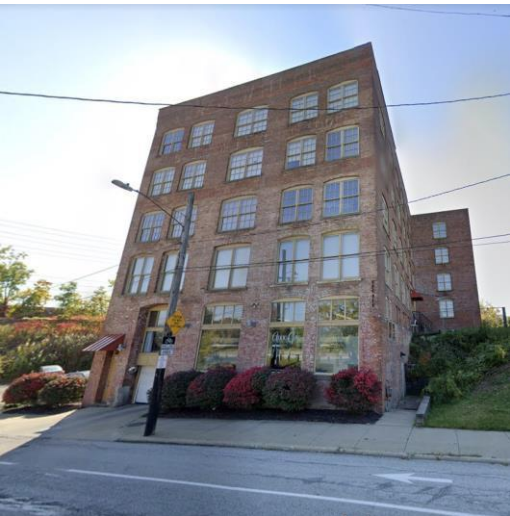
Chicle Apartments, 10307 and 10335 Detroit Avenue
