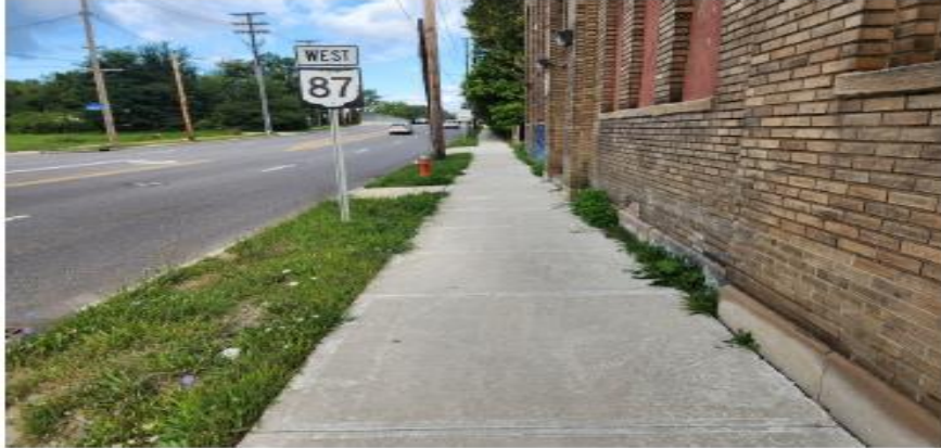
View northwest at the front of the structure on Buckeye Road.
