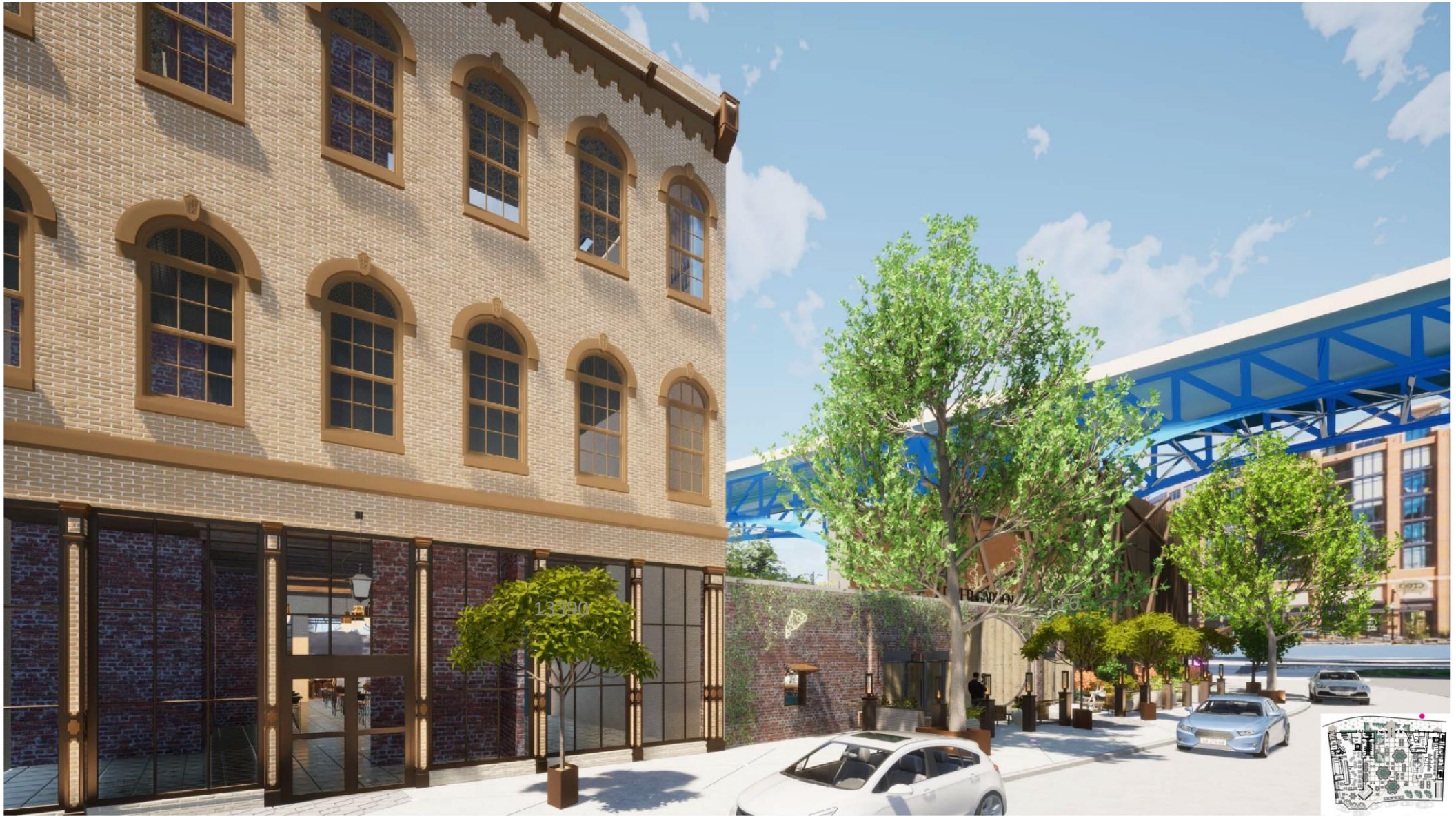
STREET VIEW SOUTH
