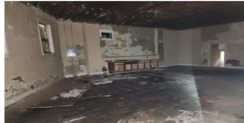
View of a typical first floor room.
