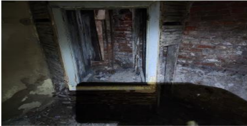
View of the dumbwaiter elevator shaft and piping in the basement.
