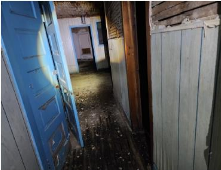
View of a typical second floor room.
