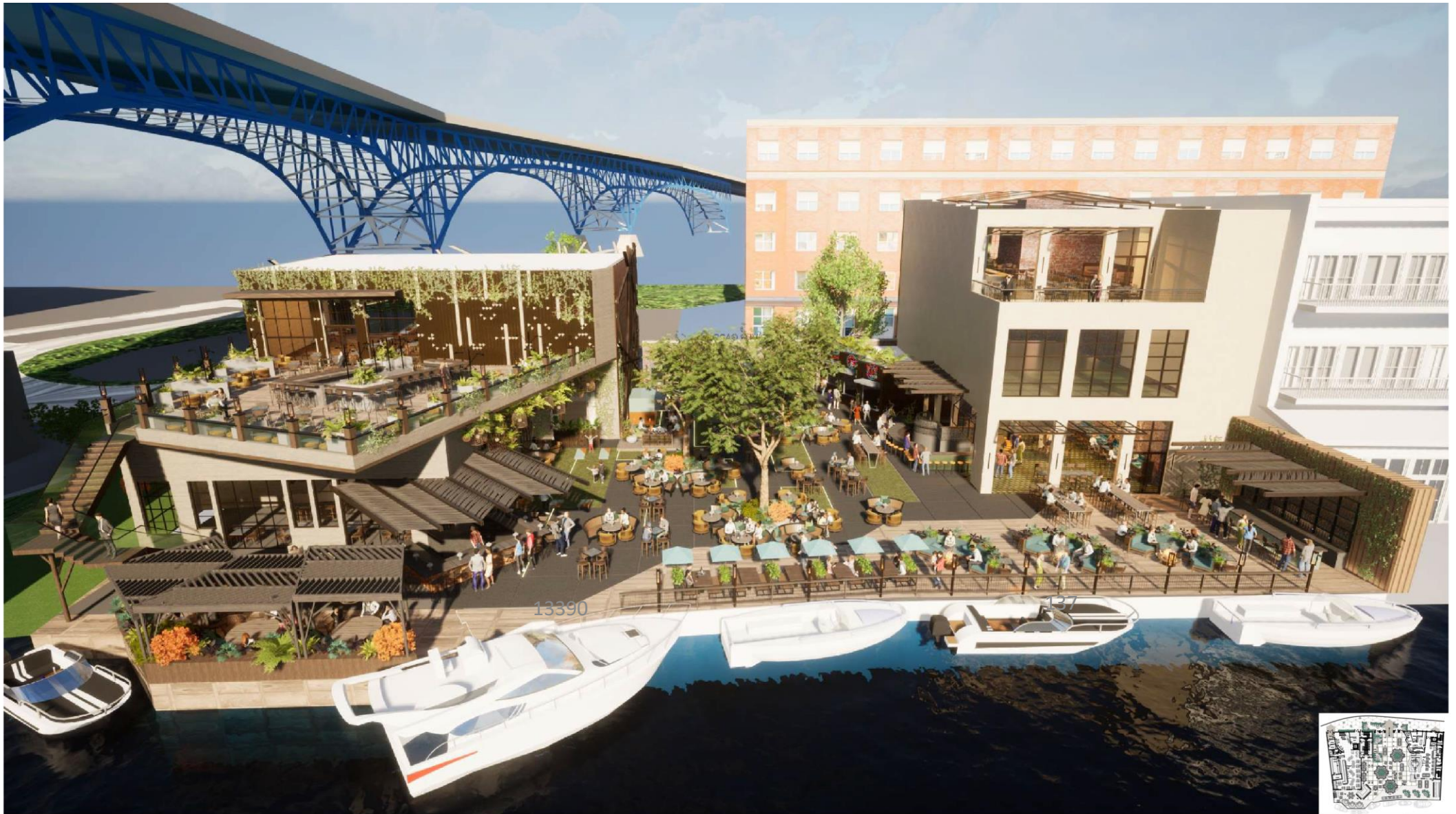
OVERALL VIEW FROM RIVER
