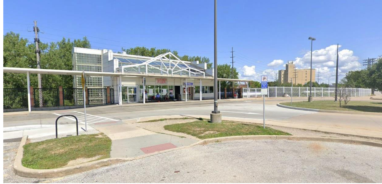
RTA West Boulevard - Cudell Station, 10108 Detroit Avenue
