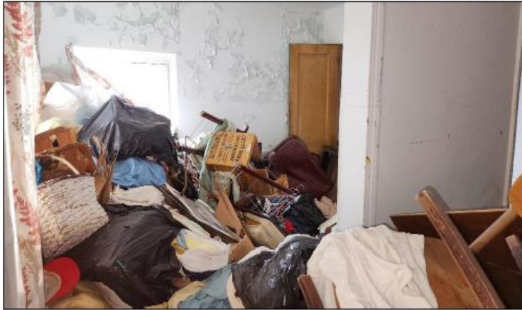
Photo 3: Interior view of Subject Property building.
