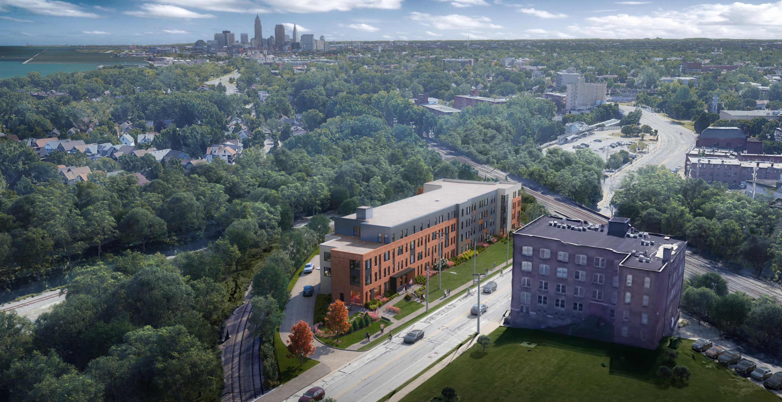
Depot on Detroit | Overall Project View
