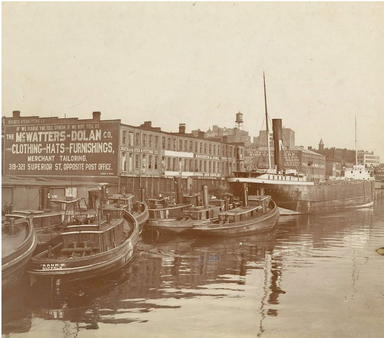
VIEW FROM RIVER C. 1903 THE HAUSHEER AND SONS BUILDING
