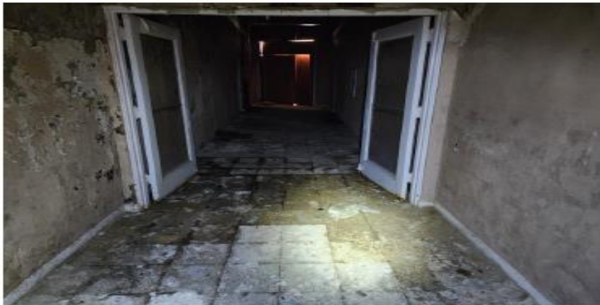
View of the entry hallway on the first floor.
