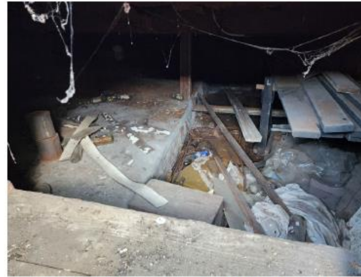
View of the storage space under the stage area.
