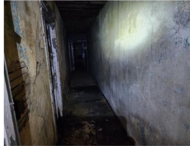
View of the second floor hallway.
