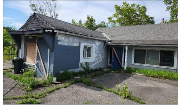
Photo 2: Eastern side of rear Subject Property building.
