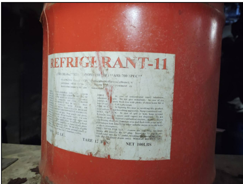
18 : 18 Multiple containers of Refrigerant-11 on floor near chiller. Contains trichlorofluoromethane a solvent/CFC. Worldwide production of CFC-11 was banned as of 2010. Health hazards include central nervous system impacts.
