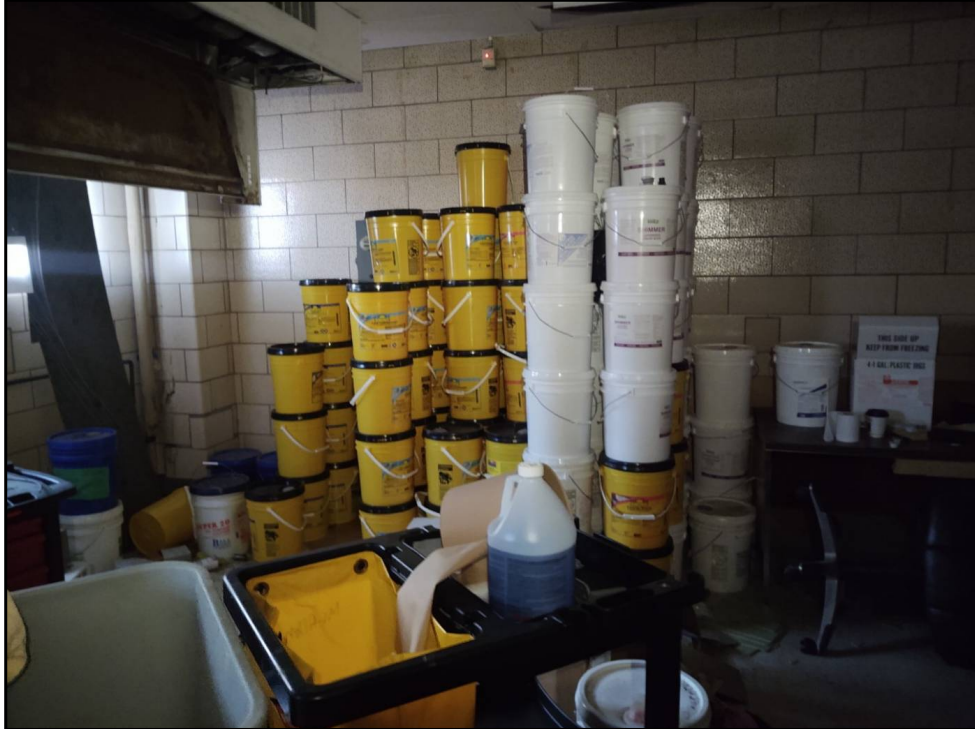
9 : 9 Custodial area. Cleaning products are appropriately stored. De minimis quantities of harsh cleaners and strippers properly stored in cabinets.
