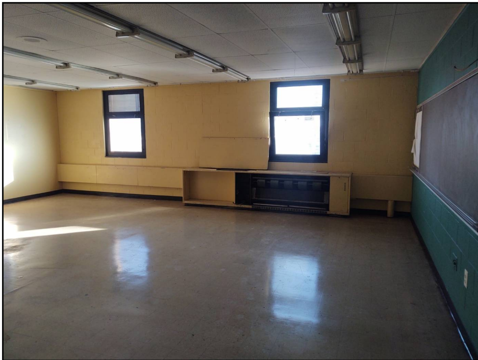
30 : 30 Representative view of third floor classroom.
