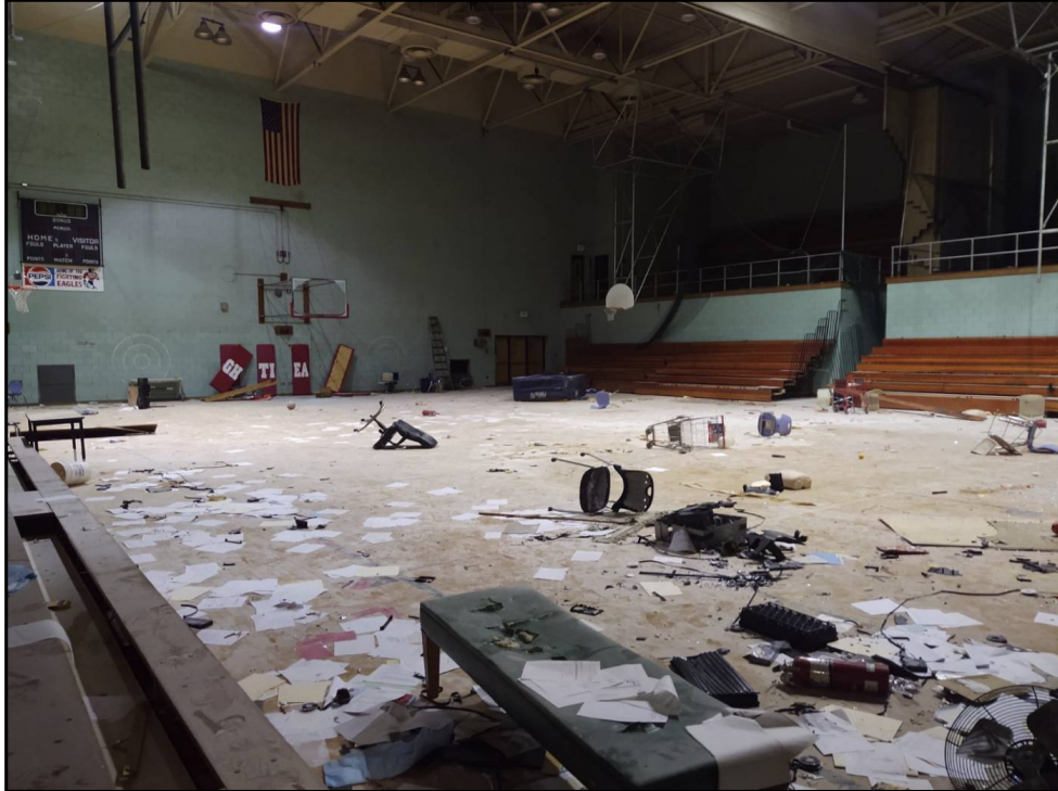
7 : 7 View of gymnasium. Vandalism apparent.
