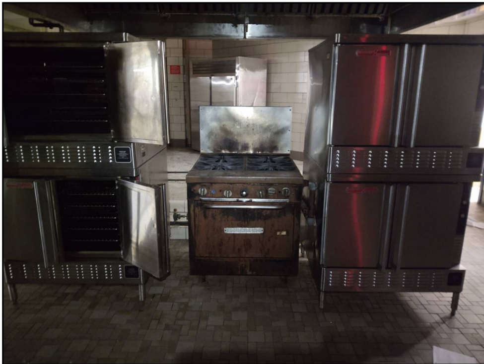
26 : 26 View of industrial kitchen equipment. Grease trap was not observed, but may still be present.
