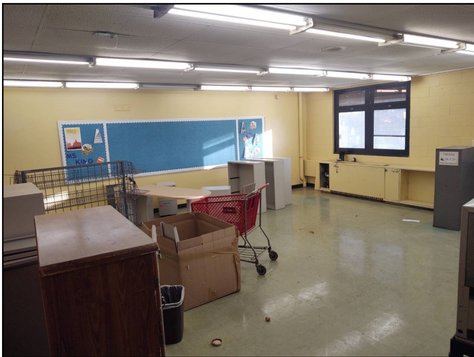
4 : 4 Representative view of first floor classroom. Vandalism damage is minor, compared to other classrooms.
