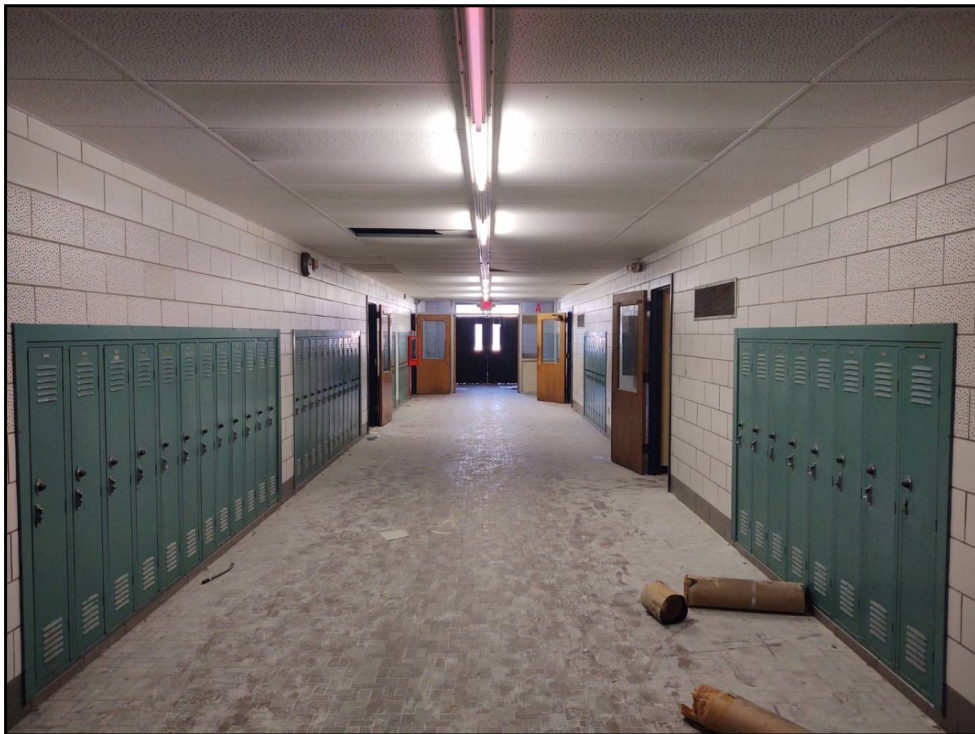
2 : 2 Representative view of first floor hallway.
